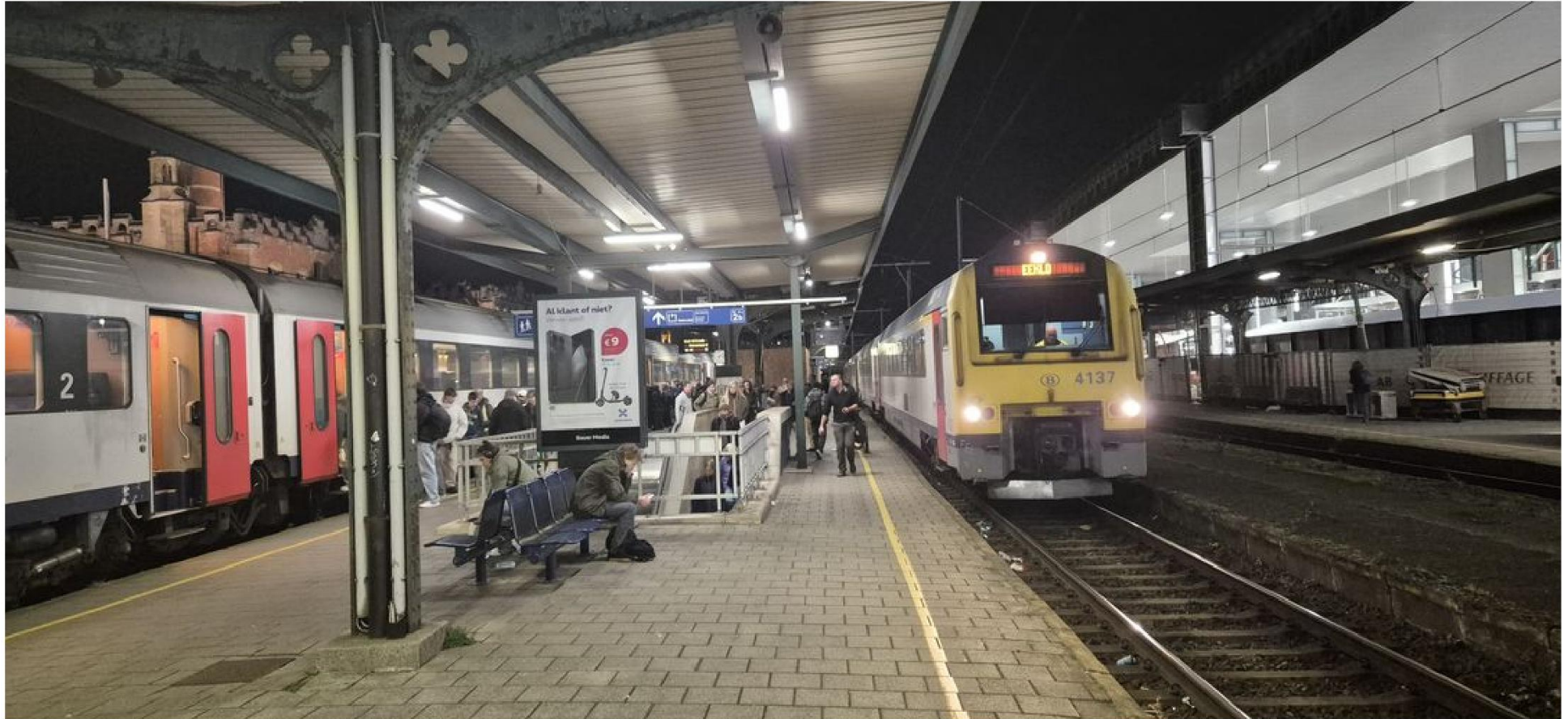
The three remaining 1913 platforms at Gent St. Pieters have not long to go now as the next set of new platforms are nearly ready. Here is a busy scene on the 4th November 2025. Photograph by Iain Dobson
