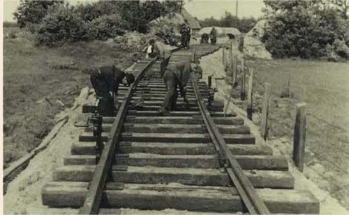
Construction of the railway connection at Camp Westerbork Wikipedia
